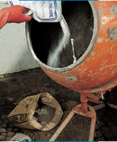
Preparing waterproof mortar admixed with Idrosilex Powder
