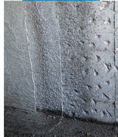
Applying mortar admixed with Idrosilex over concrete roughened with a bush hammer
