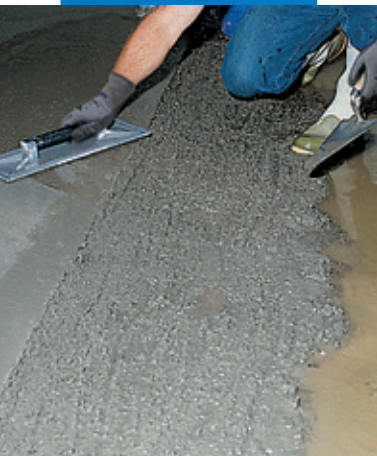
Screeding with mortar admixed with Idrosilex Liquid
